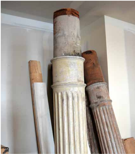
The original wood columns, some of which are load-bearing, are being restored and in some cases, portions are rebuilt.
