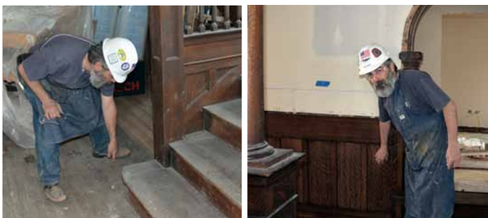
Left: Tony Frisone shows where the stair edge was cut off and will be replaced. Right: The beautiful quilting on the refinished white oak.
