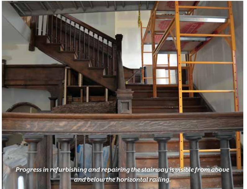
The original wood columns, some of which are load-bearing, are being restored and in some cases, portions are rebuilt.
